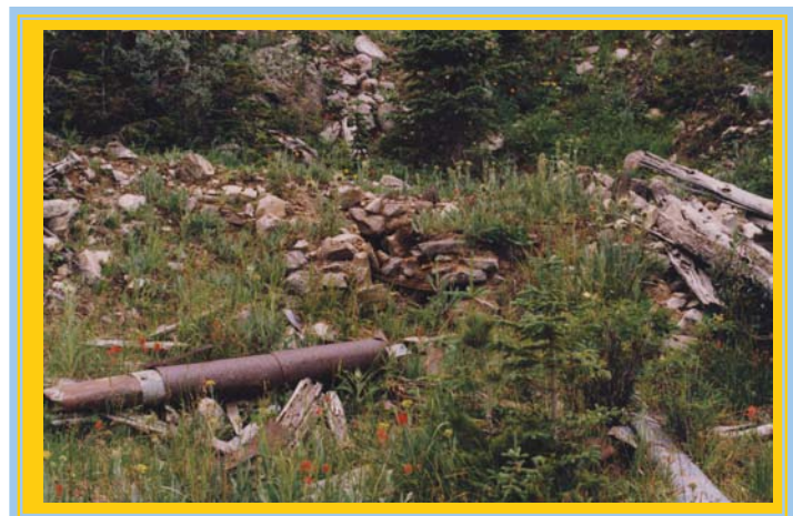
↑ The stovepipe for the ventilator stove. Note the portal is completely caved in, but the rails are still showing.
