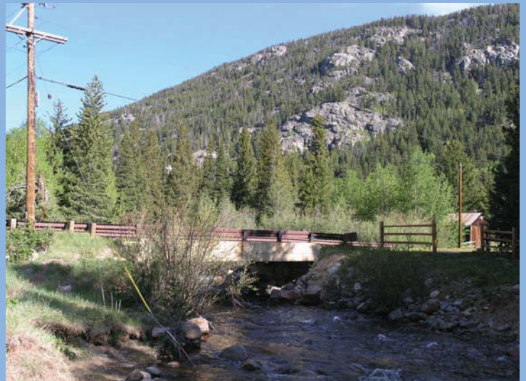
Low Flow at Sixth Street Bridge – May 29, 2012
