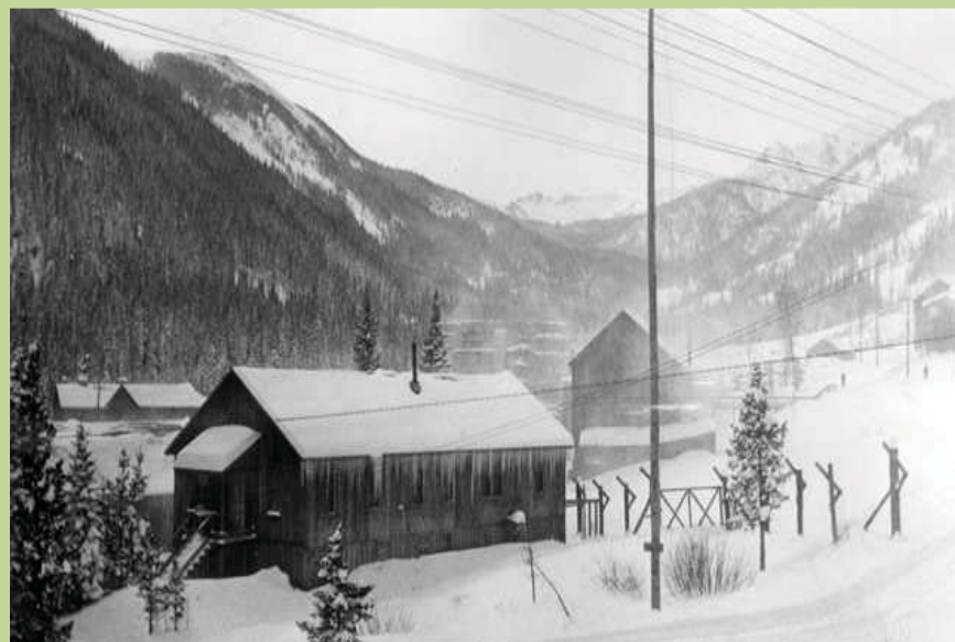
▲ East Portal dormitory for engineers/contractors December 1927
