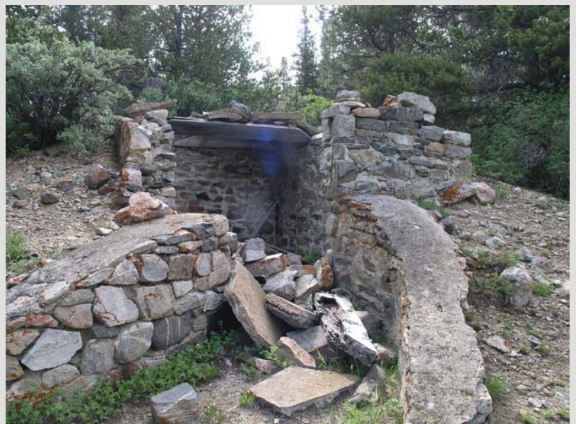
The stone housing for the Dixie Lodge generator is still visible.
