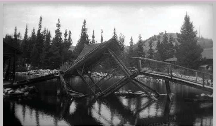
1942 – The Pagoda Bridge has collapsed. Photo by Muriel Wolle
