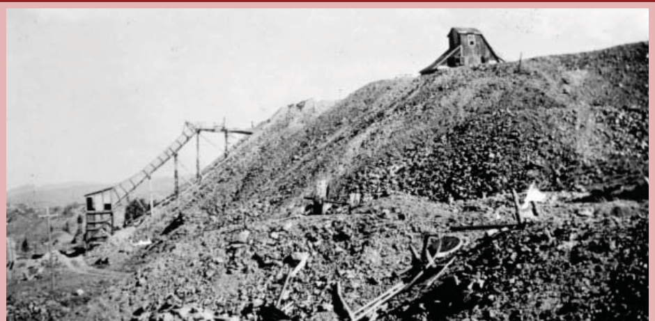
Shaft House and Loading Chute at Caribou Mine
