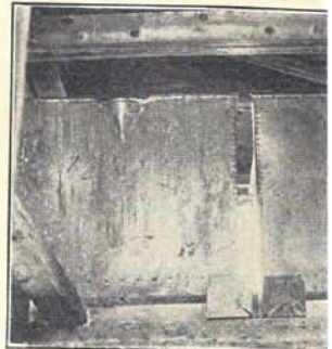
Two of the four steel tanks in of these will be used for water.
