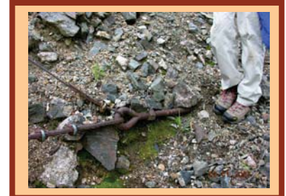
Cables secured to the ground↑
