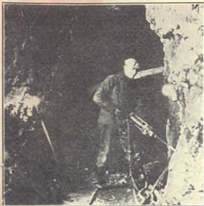
Using air drill in our mine. This man is working near where we recently struck ore that assayed $2,800.00 per ton.
