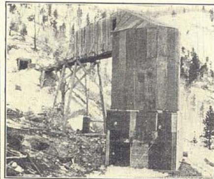
Portal of mine, trestle, upper ore bin, or bin No. 1 and tramway loading station. This bin holds seventy-five tons of ore.
