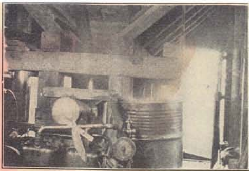
Tramway loading station, and bottom of ore bin No. 1 at mine. Also shows part of engine used to run air compressor now used at mine.
