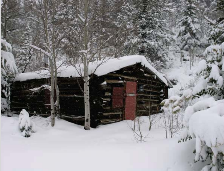
◀ This cabin at the Hessie turnoff was the Sullivan brothers' cabin that Jay used. It is also known as the Geyser cabin, built in 1878. Photo by Diane Brown
