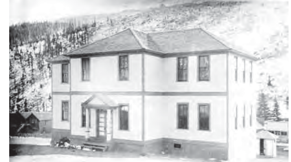
Figure 3.10. Built in 1896, Eldora's two-story, four-classroom schoolhouse may have been the most ambitious symbol of the community's boomtown hopes. It was demolished around 1939, and the materials were salvaged to build many cabins in the area. (Eldora Civic Association.)
