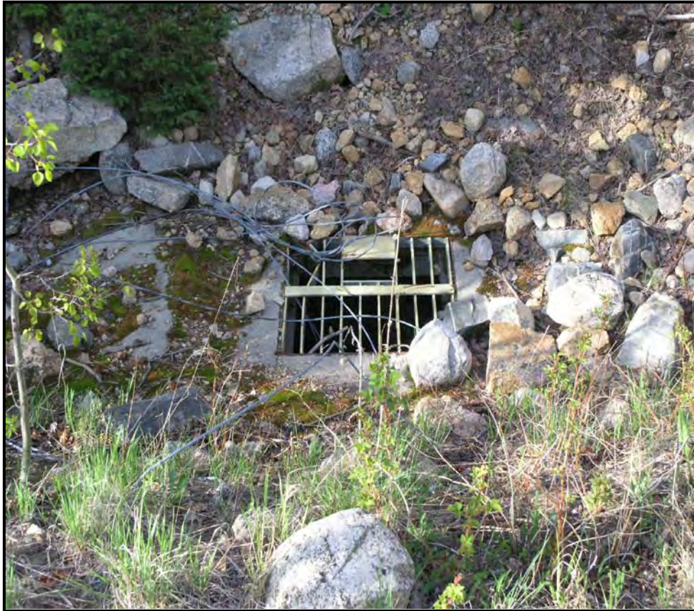
Figure 2.4. Closed Mine Shaft
